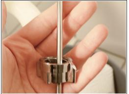
Below the sink is the pivot nut. Turn the pivot nut counterclockwise until it is completely loose and remove from the pivot rod.
