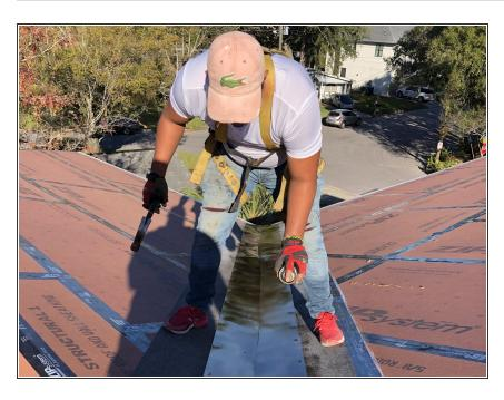
Depending on where the damaged tile is on the roof, be sure to prime underlayment before adding new roof tile on top.
