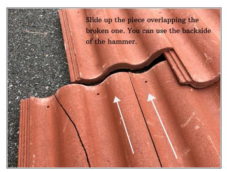
Using the backside of the hammer to slide up the piece overlapping the broken one and using a drill to unscrew any screws (which won't be necessary if you're using roof cement). Replace the tile with the new one and glue in place.
