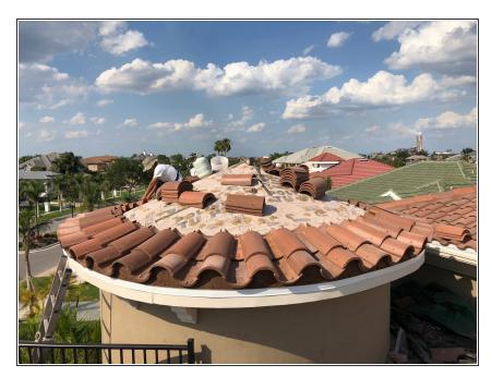
Be sure to use affective safety harness when operating in unsafe conditions. Carefully remove the damaged tile(s) using your hammer & crow bar.
