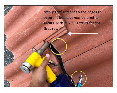
This is an initial point of view for replacing a single broken tile. You can see the application of roof cement in the crevice of the tile. To reassemble your device, follow these instructions in reverse order. Number one thing of importance is your safety, my goal is for this guide to give you a general idea of the steps it takes to construct/repair/replace a tile roof.
