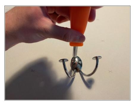
With your screwdriver, continue screwing the screws in until they're flush with the towel hook.
