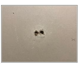
After removing the anchor screws, take your spatula and press it flush with the wall. Remove debris from the drywall to make the wall flat.
