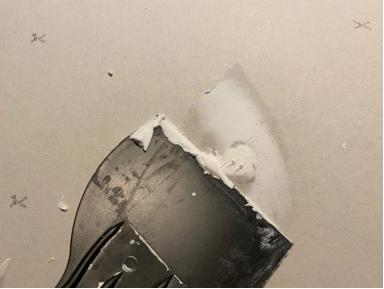
Take some patching and with your spatula, apply it on and around the holes in order to fill it up to the surface of the wall.
