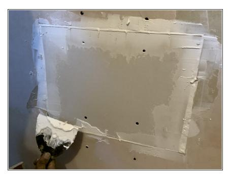
Apply drywall filler over the mesh tape and the holes left by the screws using a putty knife.
