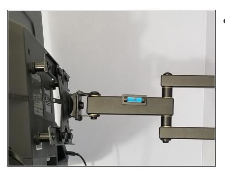
Make sure the TV is secure and well-centered on the wall mount using a spirit level gauge to confirm the inclination.
