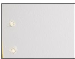
Fill the holes where the screws were secured using drywall spackle.
