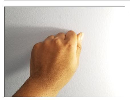
Locate the wooden studs on the wall using a stud finder or knock on the wall to see if the stud is behind the wall.
