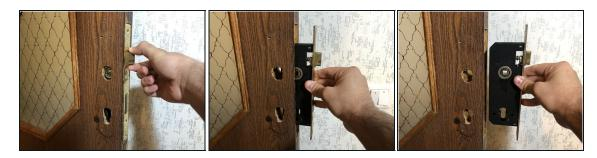
• Grasp the mortise lock on either side and pull it out from the edge of the door.
