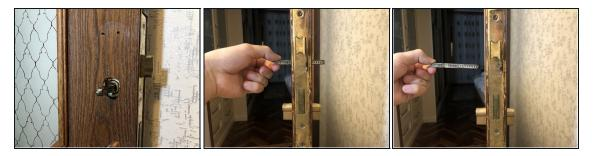
• Pull out the spindle (the rectangular piece of metal) from the door.
