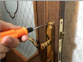
Use a flathead screwdriver to remove the eight 6 mm screws on both handles.
