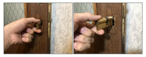
• Pull the lock cylinder out to either side of the door.
