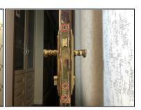
• Determine the position of the screws on both door handles and the front plate.
