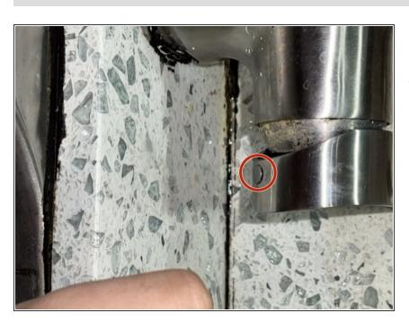
Put the rubber stud in the outer hole to cover the space and secure the screw in place. To reassemble your device, follow these instructions in reverse order.
