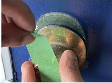
Remove the tape on both sides of the lock carefully.
