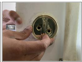
Align your new lock with the given holes on the door.
