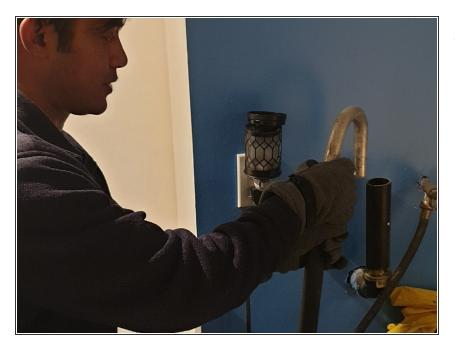
Wear proper safety gloves and remove the drain hose carefully.
