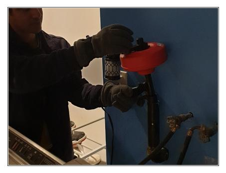
Use a snake drain and rotate the handle to unclog all the debris.
