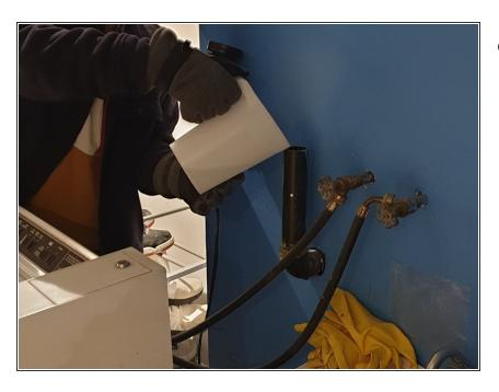
Pour hot water to help in the process of cleaning the clogged drain.
