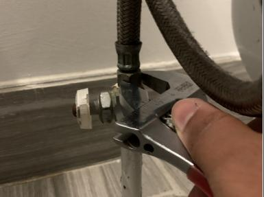
Using the wrench, disconnect the tank hose from the pipe by turning the wrench clockwise until the hose is completely disconnected from the pipe.
