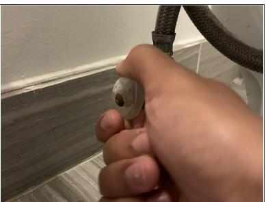
Turn the toilet shut off valve counter clockwise.
