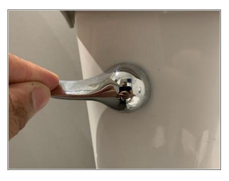
Flush the toilet (the one that needs the valve to be replaced).
