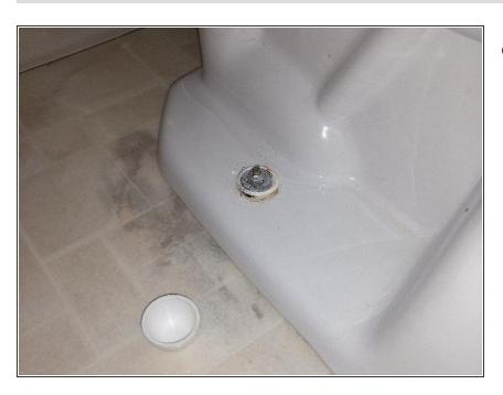
Tighten the nuts and bolts on each side of the toilet and replace the bolt-protectors.
