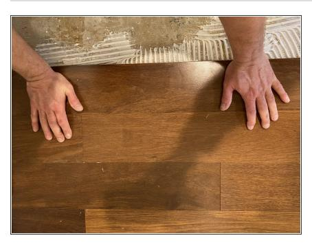
Carefully place the boards on top of the glue, making sure to push the seams of the planks together.
