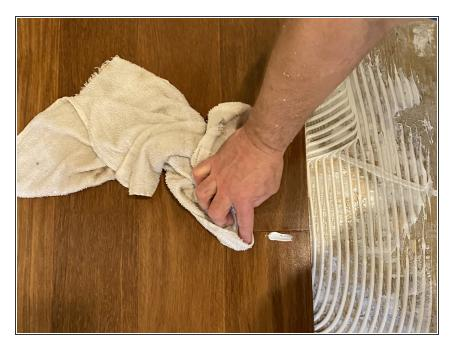
Some of the adhesive may come through the seams, so wipe off any excess glue with a wet rag.
