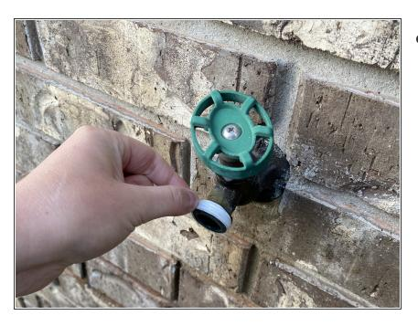
Using plumbers tape, wrap around the spigot once ensuring that is it fully covered.
