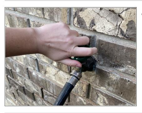
Turn on water to ensure there are no leaks/water sprays.
