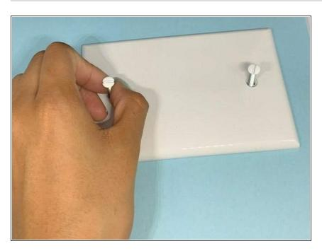
Insert two screws into the holes of the new wall cover.
