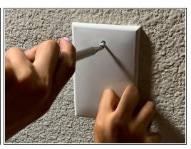
Tighten the two screws with a flathead screwdriver.
