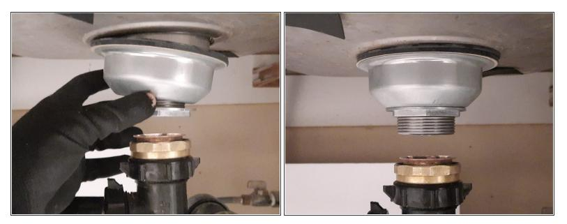
• Tighten the lock nut under the strainer with your hands.
