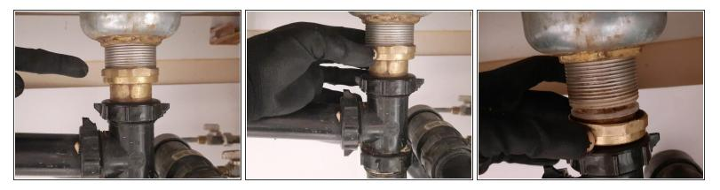
Loosen the bottom lock nut under the sink with your hands. If your hands are not enough, use a 12" pipe wrench to loosen the bottom nut out.
