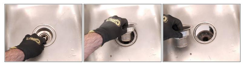
(i) The top strainer easily comes off now due to no nut holding it in place.
