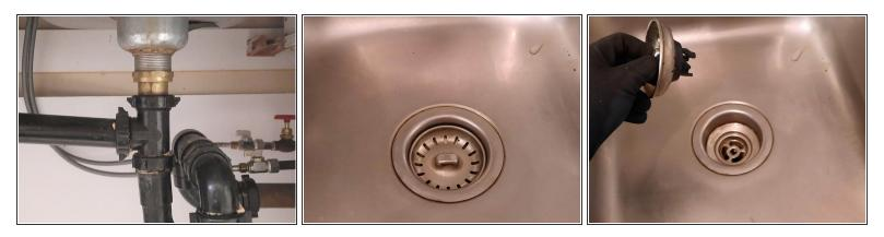
Inspect the strainer under the sink and inspect the basket over the sink. Take out the basket from the top.
