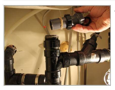
Slide the old trap adaptor nut and nylon slip washer over the tailpiece.
