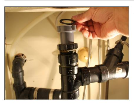
Install the tailpiece into the trap adaptor with the tailpiece washer inserted on top.
