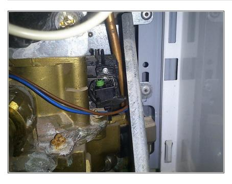
Put it back, reconnect mains but keep an eye on the gas flame that might turn on without the switch is being pressed (if it is so the switch is not dry inside). Say thanks to me ( atosmaximus (at) gmail.com :-) To reassemble your device, follow these instructions in reverse order.
