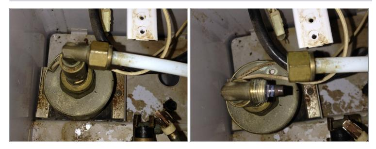
• At the top of the water pump, there is a high pressure teflon hose that needs to be unscrewed in order to free the pump.
