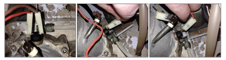
• Still not done with labelling and pulling off connectors, this time at the back of the boiler.
