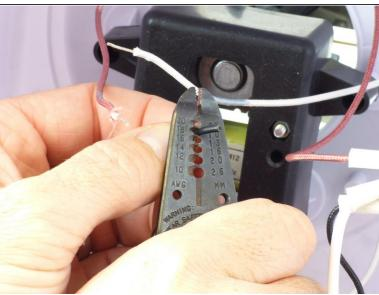
• Using the wire stripper, remove 1/2 inch of the wire insulation at the end of each wire to expose the bare wire for re-connection.
