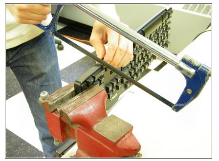
Fasten the top part of the keyboard and take the hacksaw to it. Cut off the numerical keypad part. Do not use power tools because you may produce toxic fumes and even activate fire alarm.
