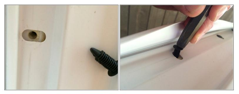
I removed the old fasteners by cutting the heads off with diagonal side-cutter and pushing the stems into the holes with a blunted nail. I pushed the new fasteners in with the back of a centerpunch.
