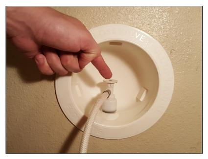
• Turn off or push down off water main valve from the wall.
